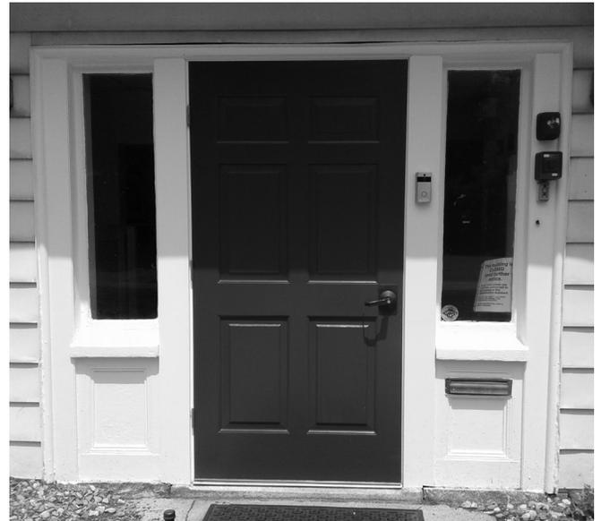
The door on Cross Street has been replaced! The frame needed quite a bit of work before it could be hung on the new hinges, as there was a large gap and rotted wood between the door and the windows. A fresh coat of paint was applied to the surrounding woodwork and it just looks great. The staff has noticed a big difference in how the door closes!
